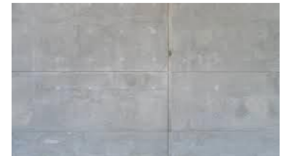
OFFFORM CONCRETE COLUMNS, BLADES, WALLS, SLAB EDGES,
