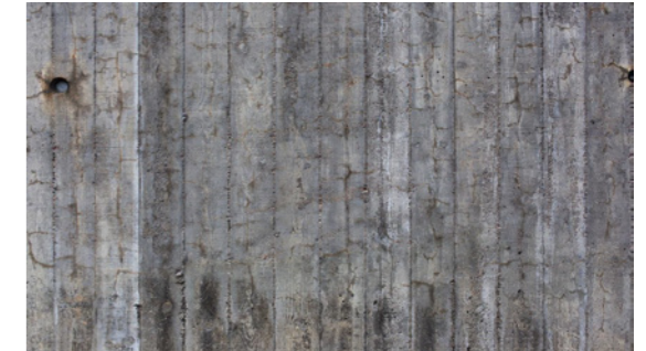
OFFFORM CONCRETE COLUMNS, BLADES, WALLS, SLAB EDGES,
